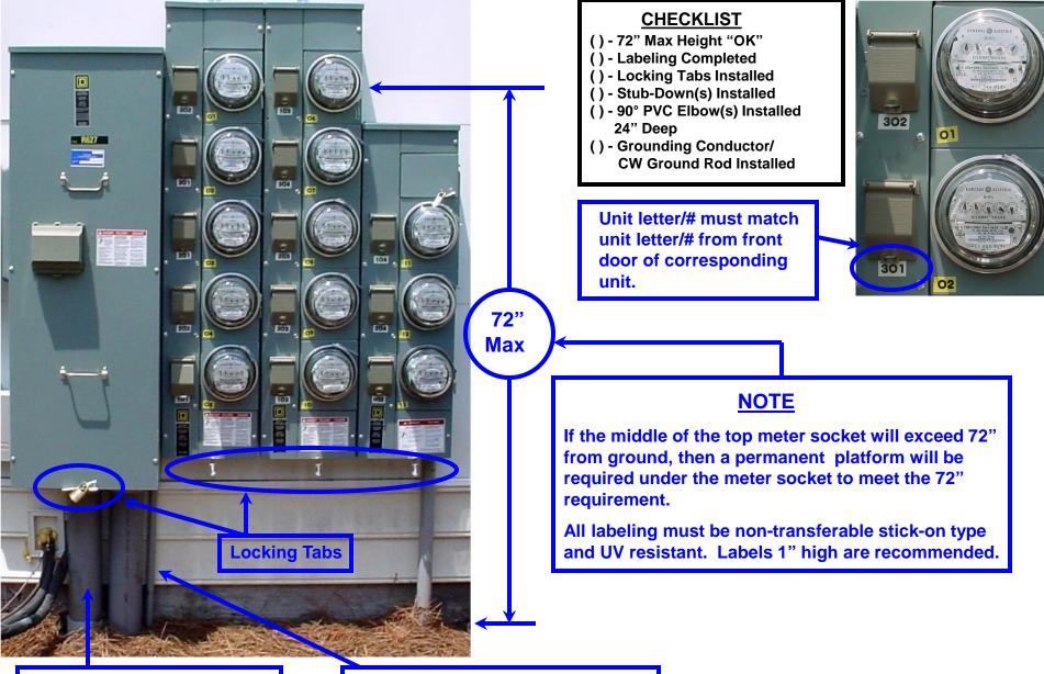
PVC stub-down with 90° elbow 24" deep Note – Contact Area Engineer for size and quantity Ground wire must be in conduit and connected to 10' x  $\frac{1}{2}$ " Copperweld ground rod.
